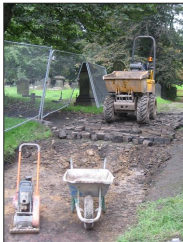
Day one on re-laying Anglican Walk
